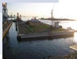
Megafloat for cooling water tanks
